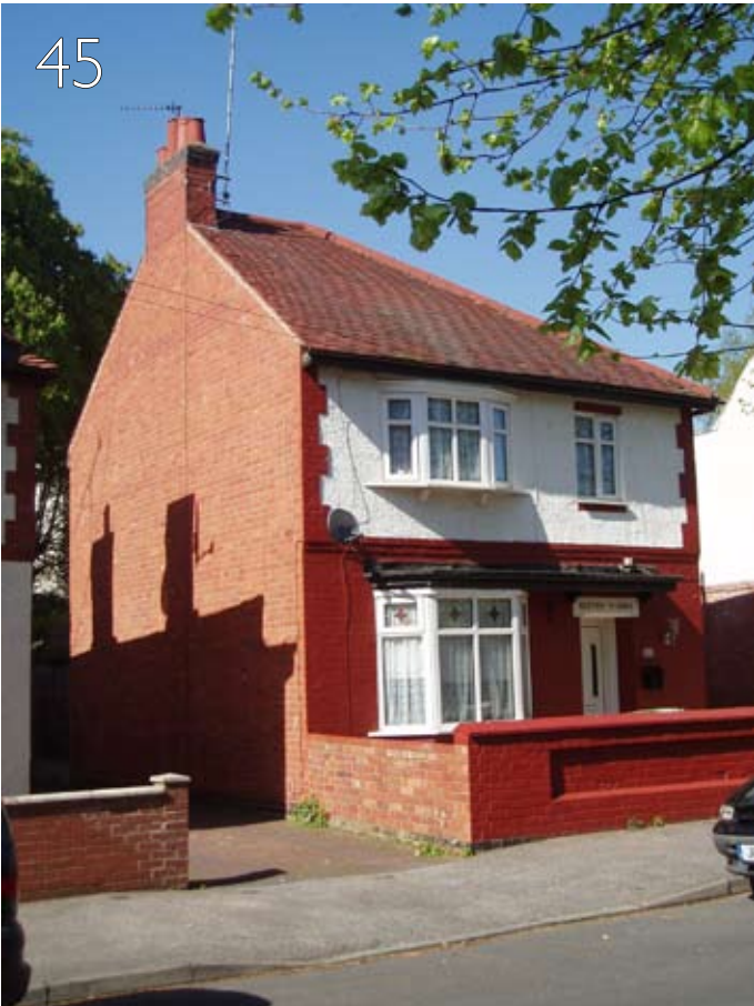
55 Earls Road built as the half of a pair that was never completed
