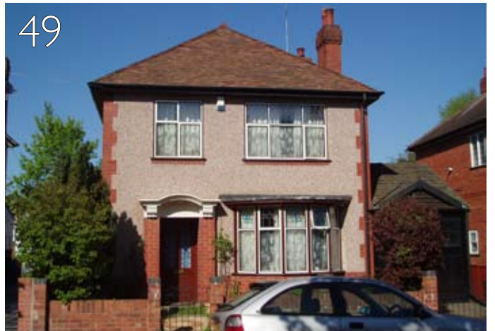
9 Earls Road 1929 by JB Hingley
