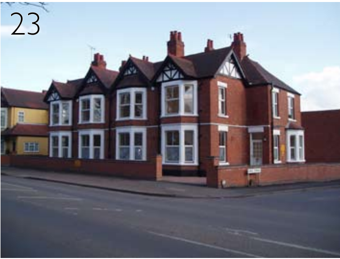
102-4 Manor Court Road c.1905. By local architect RH Smith for local developer A W Rose
