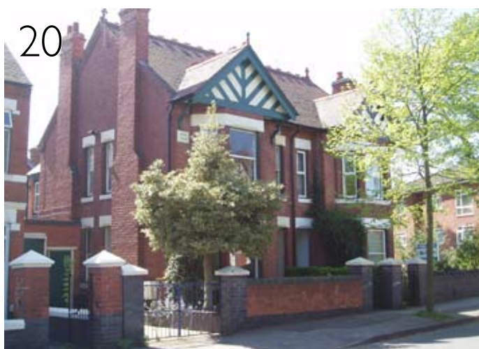
Lyndhurst and Milton Villas, 157-9 Earls Road. Built 1897 for Ernest Voules a tile manufacturer's clerk
