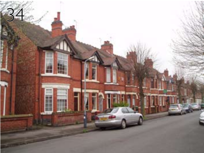
10-12 Earl Street, South West Side. Smaller semi detached houses stand close together in the north eastern arm of Earl Street
